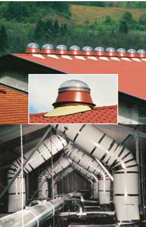
N. 14 SOLARSPOT 650, of very complex configuration, made of 22 tubular sections, light 560 sqm of the enlarged workshop FRE.TOR in Puos d'Alpago, Belluno (Italy). (2001)
